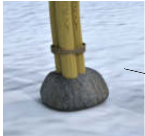
footing via traditional Asian stone and bamboo resting connection
